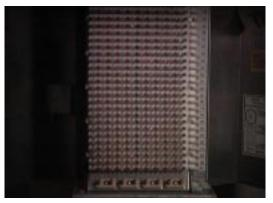
(a) The bottom of a phone company "crossbox" that connects customer phone lines to company wiring. The terminals in half of the box are connected to phone company wires, and those in the other half are connected to subscriber lines. No wires are connected in this picture.
