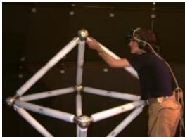
(a) A worker using the ARC system to construct a space frame.
